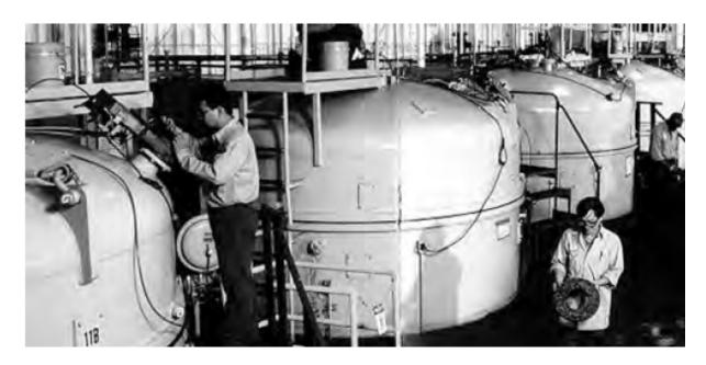
Residence time in the CVD furnaces can be days or even weeks. During this process, carbon is deposited onto the fibers and make a solid disk.
